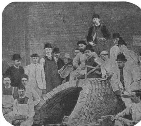
VAULT FORMED WITH SLANTING ARCHES.
