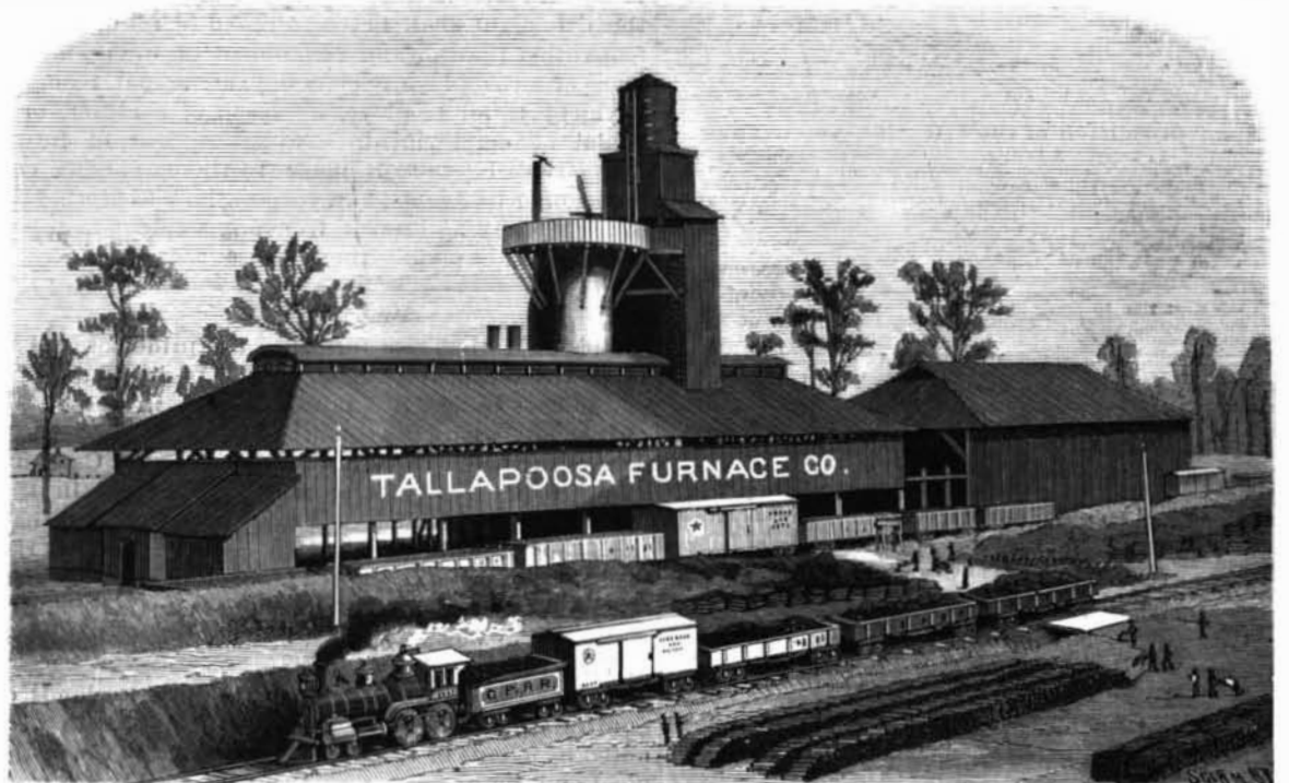
Fig. 2.—TALLAPOOSA BLAST FURNACE—CAPACITY, 50 TONS A DAY.
