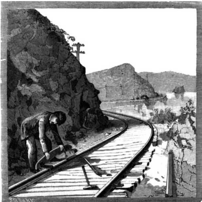
Fig. 1.—LANDSLIDE—TRACKMAN PLACING PORTABLE SAFETY STOP IN POSITION.
