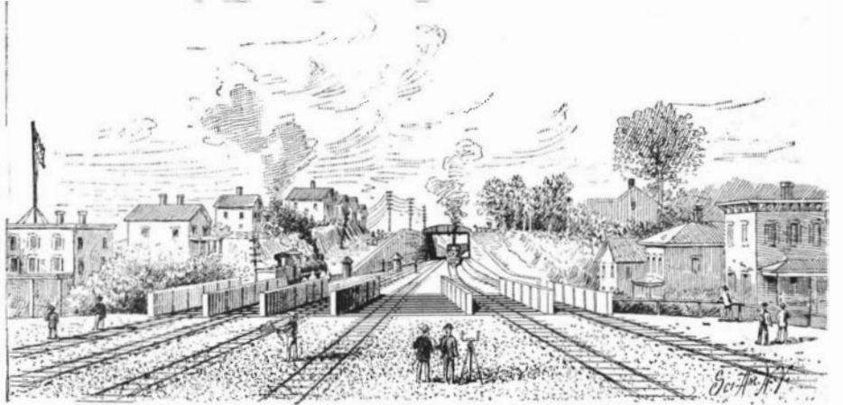
PORTCHESTER—LOOKING WEST FROM STATION.
