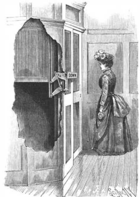
HAYWARD'S INDICATOR FOR PASSENGER ELEVATORS.
