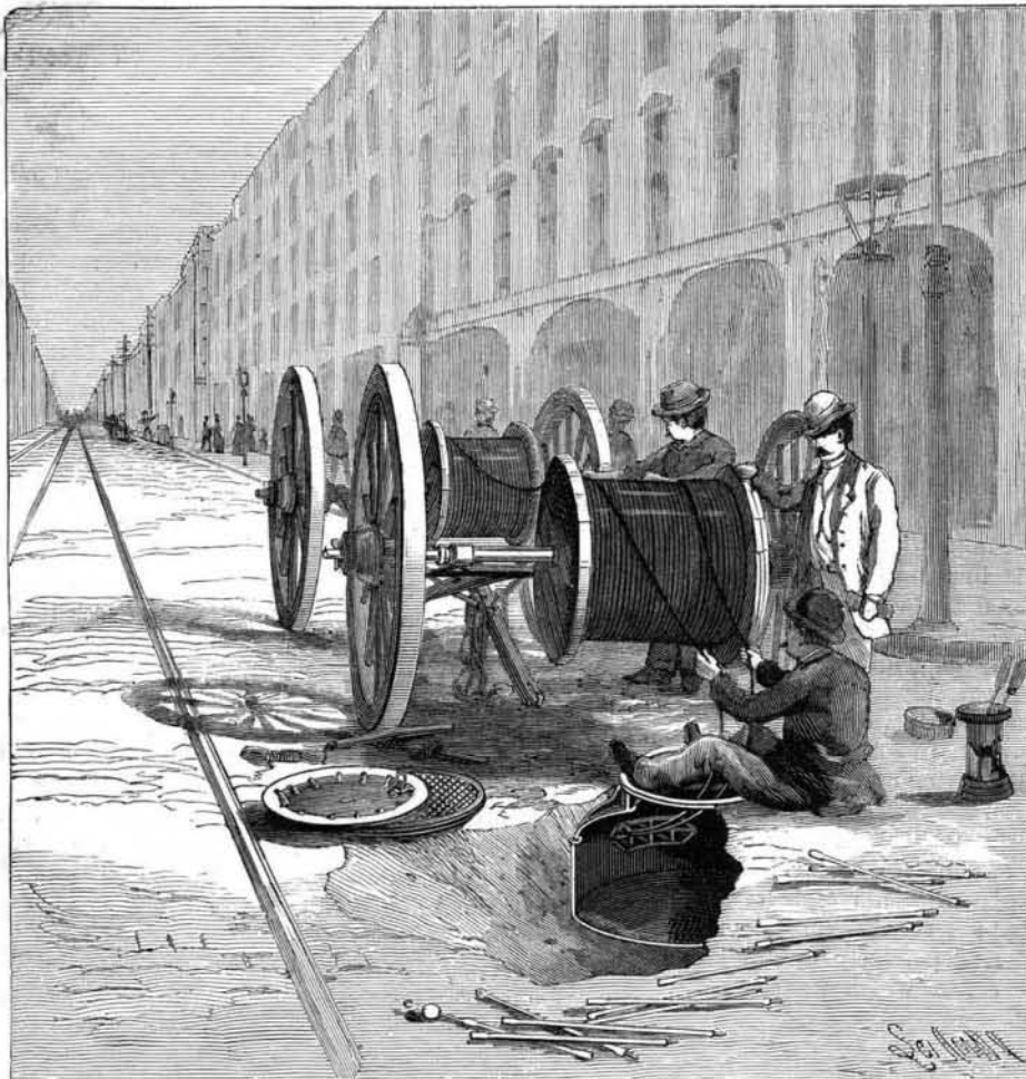
Fig. 2.—FEEDING ELECTRIC LIGHT CABLES INTO THE DUCTS OF THE SUBWAY.
