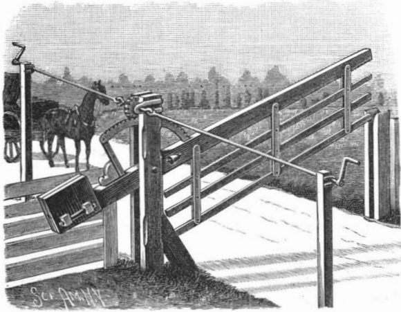
BROAD'S VERTICALLY SWINGING GATE.
