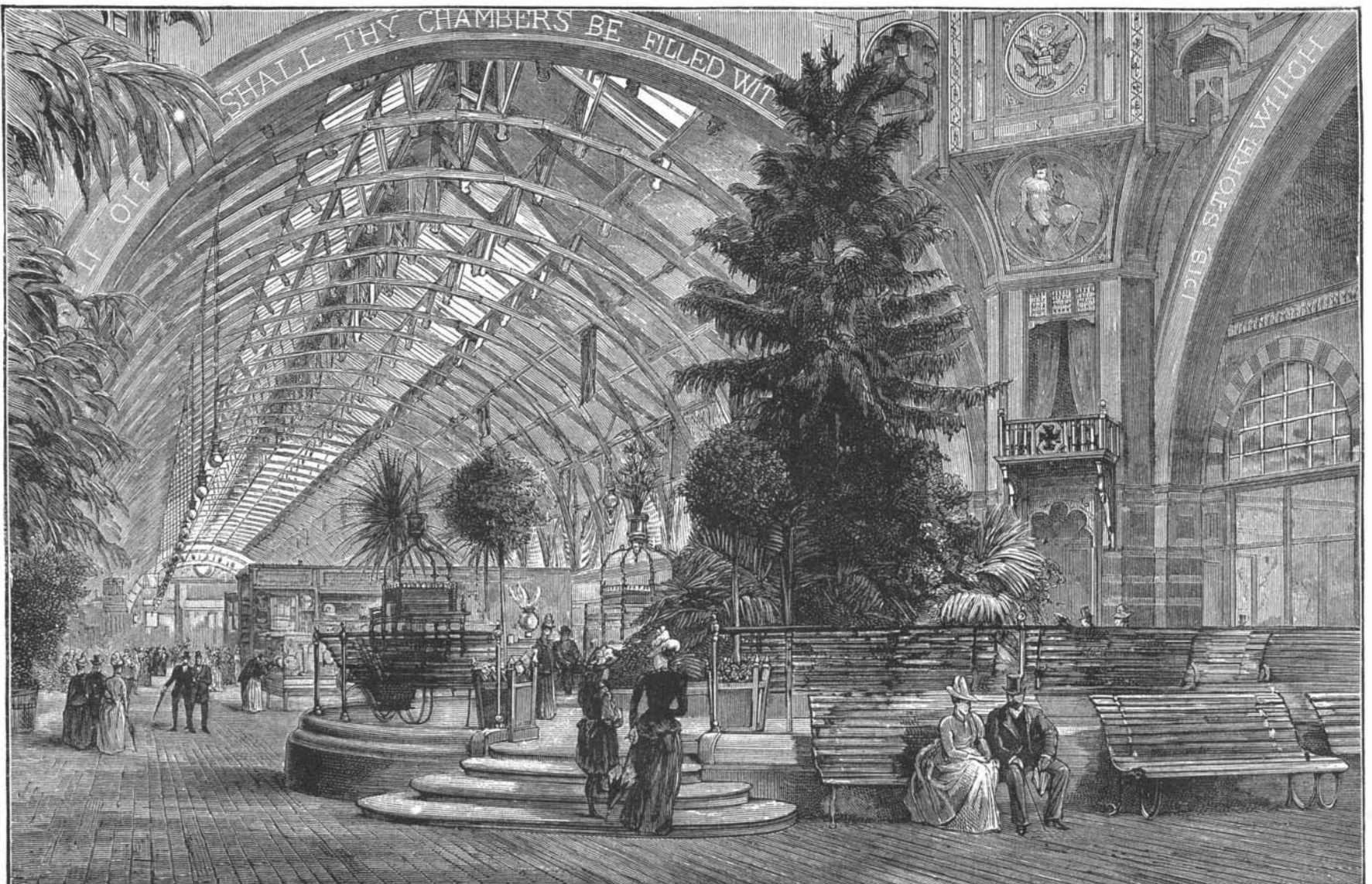
THE GLASGOW EXHIBITION—VIEW FROM UNDER THE CENTRAL DOME.
