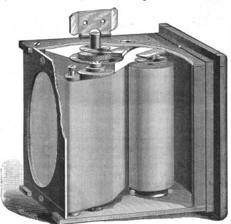
Fig. 2.-SUPPLY BOX OF THE KODAK CAMERA.
