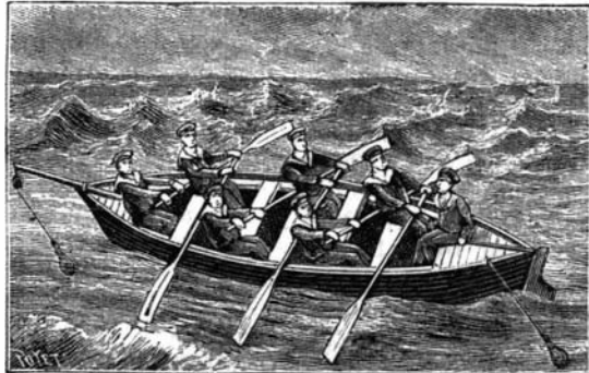
Fig. 2.—LIFE-BOAT WITH OIL BAG.
