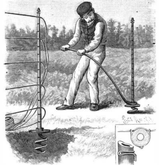
GUILLE'S METALLIC FENCE AND FENCE POST.
