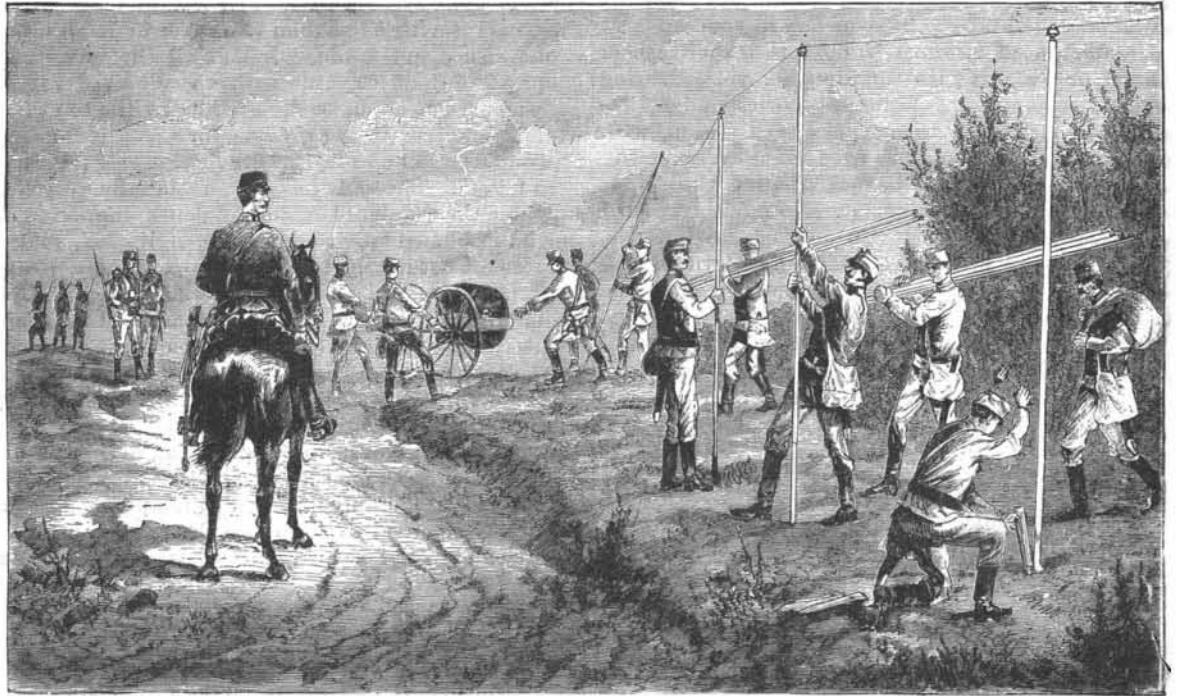
ERECTION OF THE TELEGRAPH BY THE RAILROAD AND TELEGRAPH REGIMENT.
