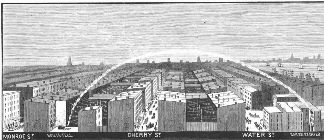
FLIGHT OF THE BOILER.
