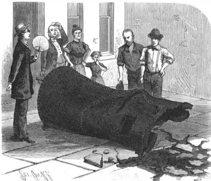
THE EXPLODED BOILER.
