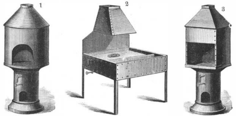
EHRGOTT'S IMPROVEMENTS IN PORTABLE FORGES.
