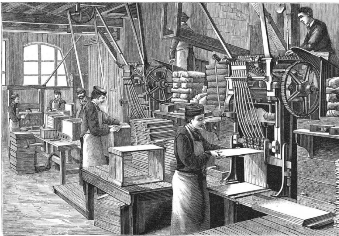
Fig. 2.—NAILING MACHINES IN OPERATION.
