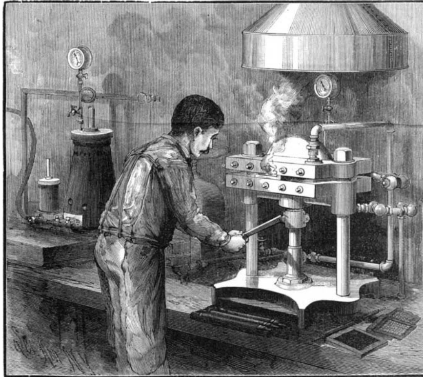
Fig. 7.—VULCANIZING TYPE PLATES AND RUBBER ROLLS.
