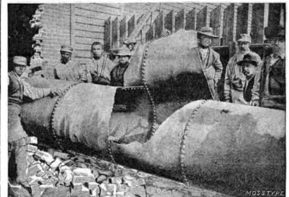
THE EXPLODED DRUM.
