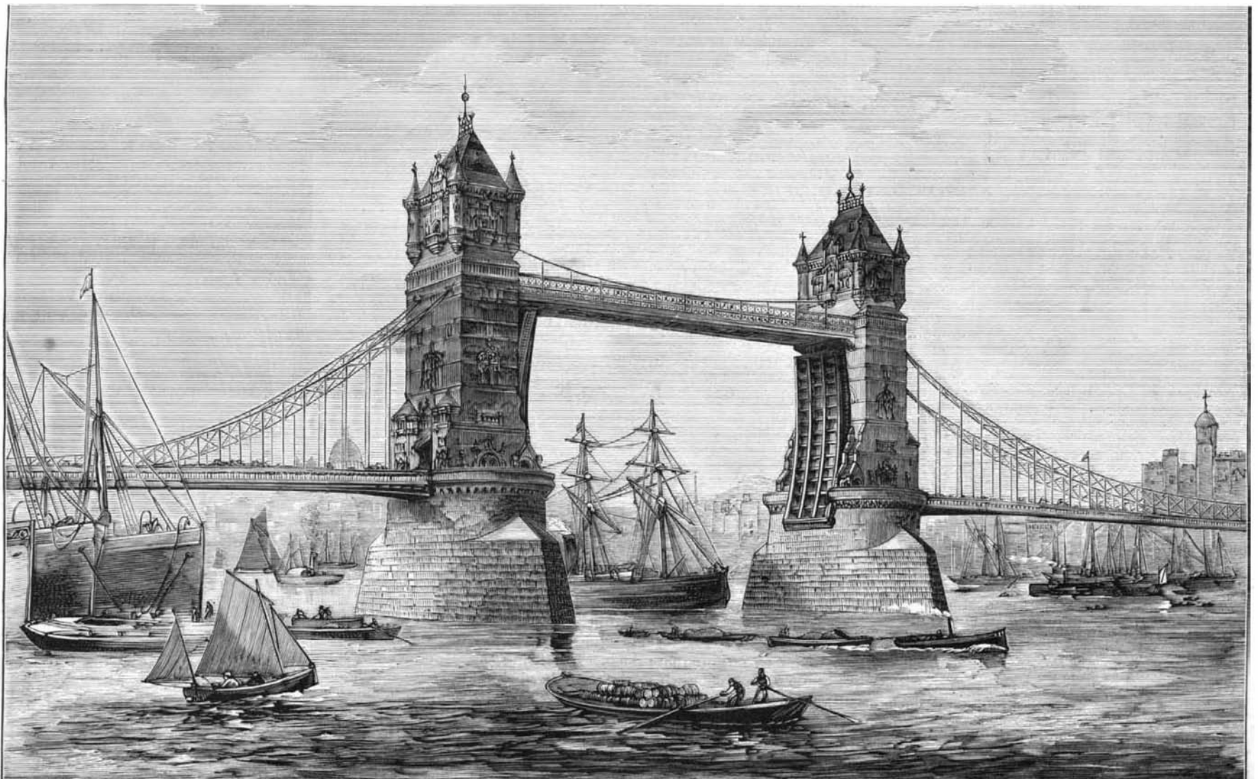
THE NEW BRIDGE OVER THE THAMES, LONDON, RECENTLY AUTHORIZED BY PARLIAMENT.—THE DRAW OPEN.—[See page 261.]
