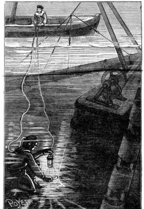
DIVERS WORKING BY ELECTRIC LIGHT.
