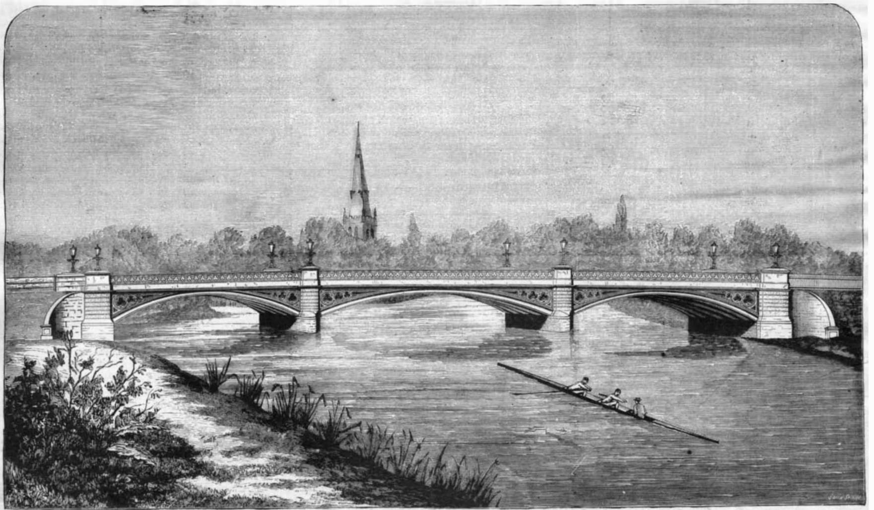
ROAD BRIDGE OVER THE OUSE AT BEDFORD.
