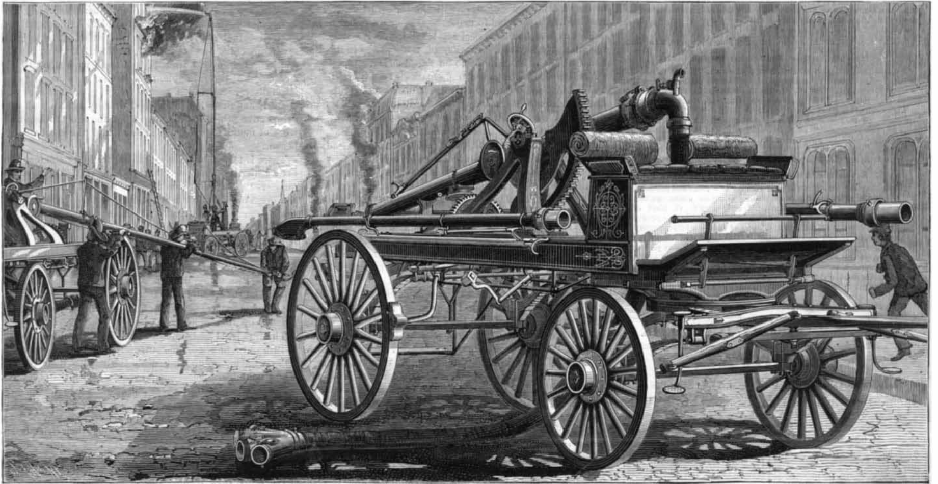
NEW YORK FIRE DEPARTMENT.—THE WATER TOWER.
