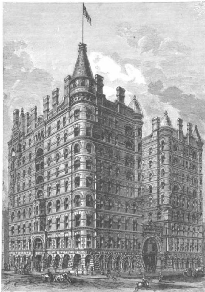
PULLMAN & CO.'S BUILDING AND GENERAL OFFICES, MICHIGAN AVE. AND ADAMS ST., CHICAGO.
