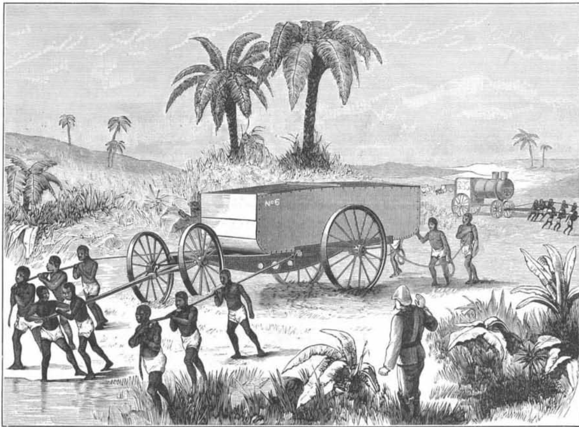
MODE OF TRANSPORTING THE SECTIONS OF THE STEAMER.
