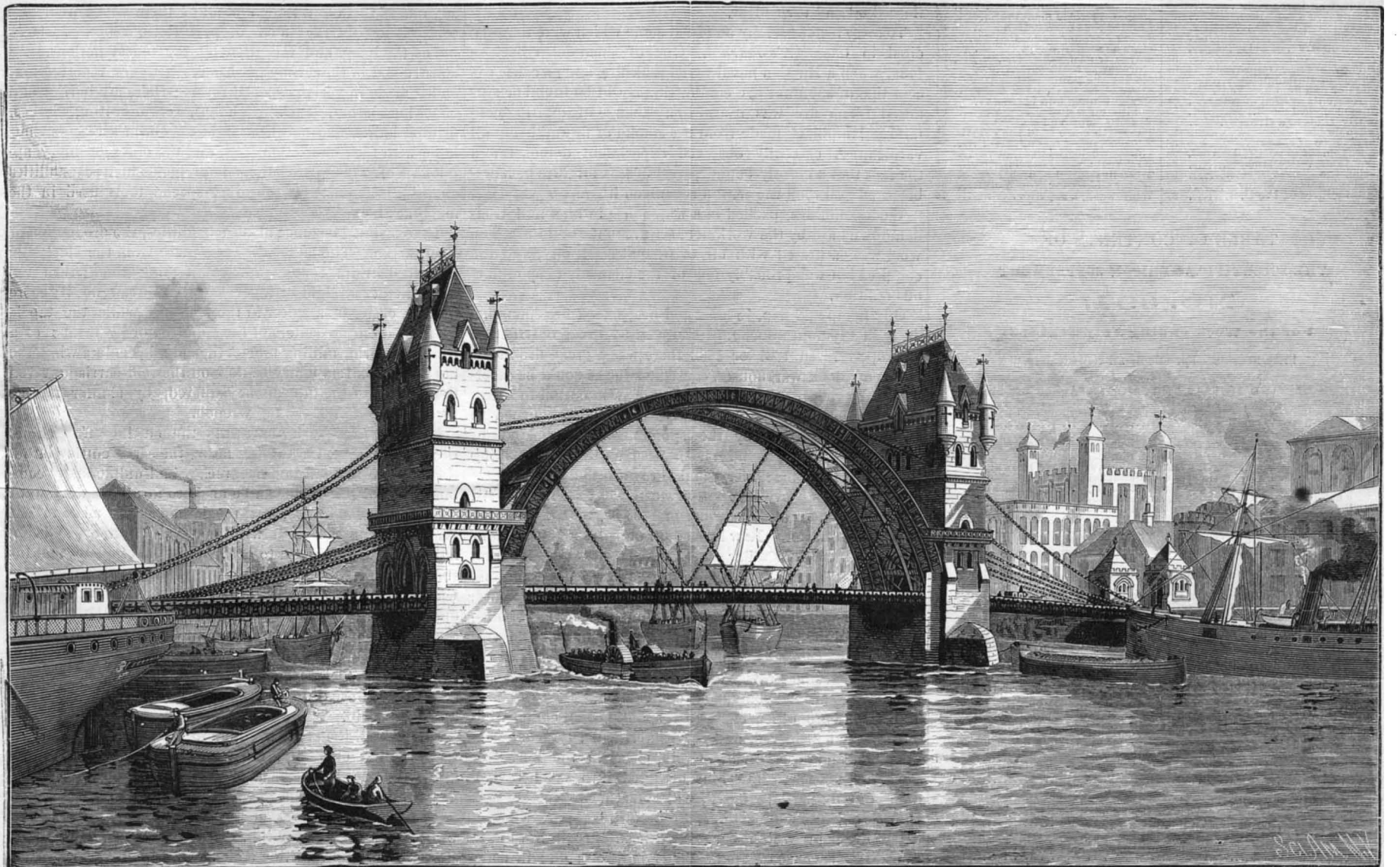
DESIGN FOR BASCULE BRIDGE OVER RIVER THAMES BELOW LONDON BRIDGE. [See page 36.]
