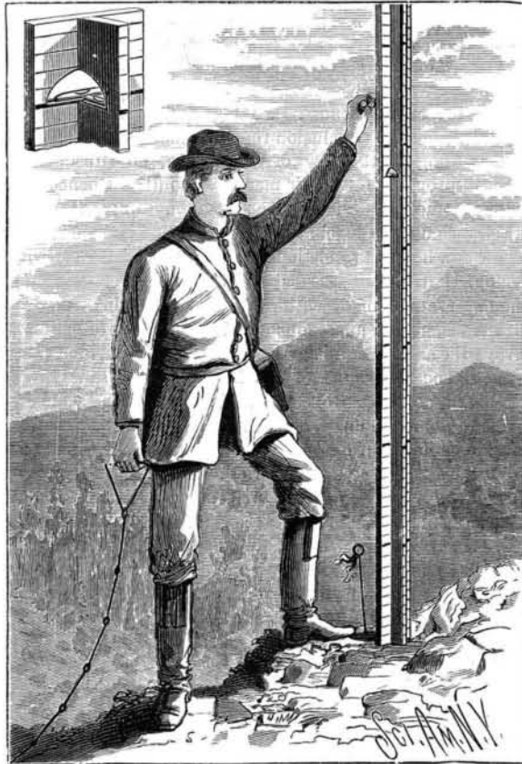
SURVEYOR'S LEVELING ROD.
