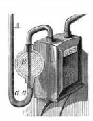
preventing the escape of gas following the destruction of the meter or the melting of the connection. Our suggestion has been heeded by Mr. Fred R. Hoard, of Providence, R. I., who has invented the simple and effective device shown in the engraving. It consists of a hollow ball, B, filled with lead or fusible metal with the exception of a central passage. This ball is inserted in the
