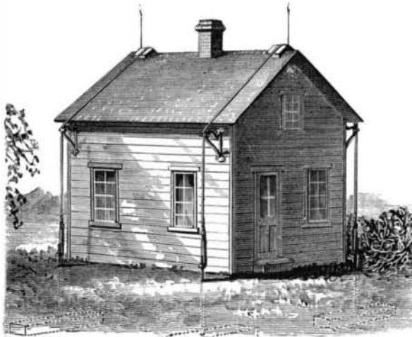
APPARATUS FOR PROTECTING BUILDINGS.
