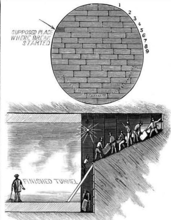
Fig. 2.—THE TEMPORARY BULKHEAD.—METHOD OF ADVANCING THE WORK.
