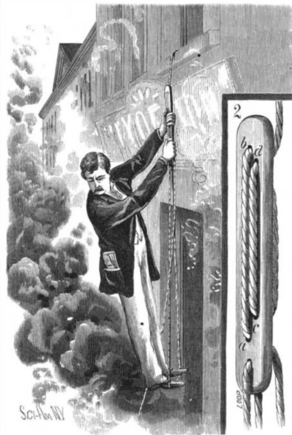
NEW FIRE ESCAPE.
