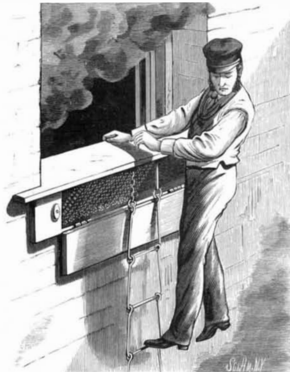
SHAW'S FIRE ESCAPE.
