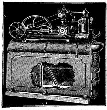
PORTABLE AND STATIONARY ENGINES AND BOILERS, 5 to 20 H.P. Return Flue Boiler, large Fire Box, no sparks. Do not fail to send for circular to SKINNER & WOOD, Erie, Pa.
