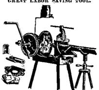
Chase's Improved Pipe Cutting and Threading Machin is the very best made for cutting off and threading Stear and Gas Pipes, Boiler Tubes, Kound Iron, Bolts, Nuts and making Stepics, from ½ to 2 inches. No pipe splitting No bevel inside or outside. No other has automatic cut off. A boy, with this machine, can do more work that two men with old systum. Send for circular. CHASE MACHINE CO., 120 Front St., New York.
