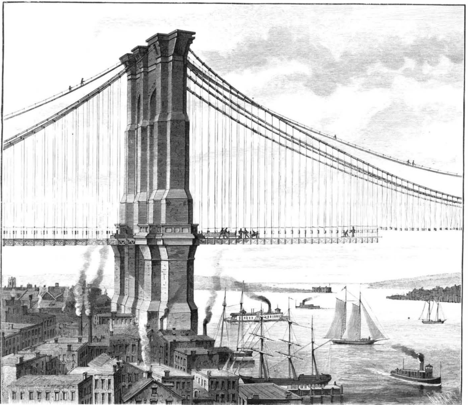
SUSPENDING THE FLOOR BEAMS OF THE EAST RIVER BRIDGE.
