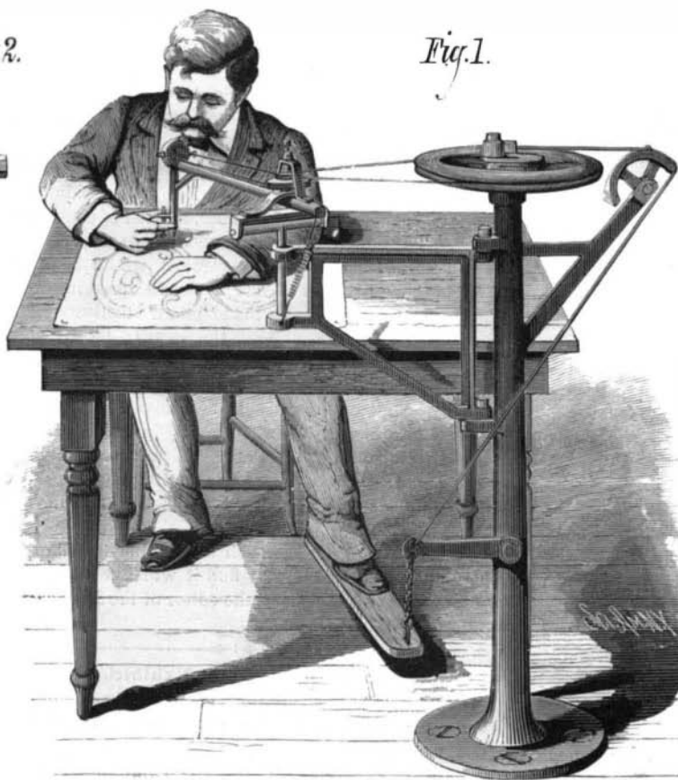
BENTLEY'S PERFORATING MACHINE.
