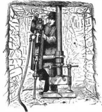
ROCK DRILL WITH COLUMN.
