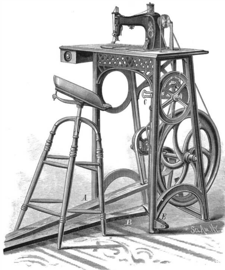
VAN WYCK'S TREADLE ATTACHMENT FOR SEWING MACHINES.
