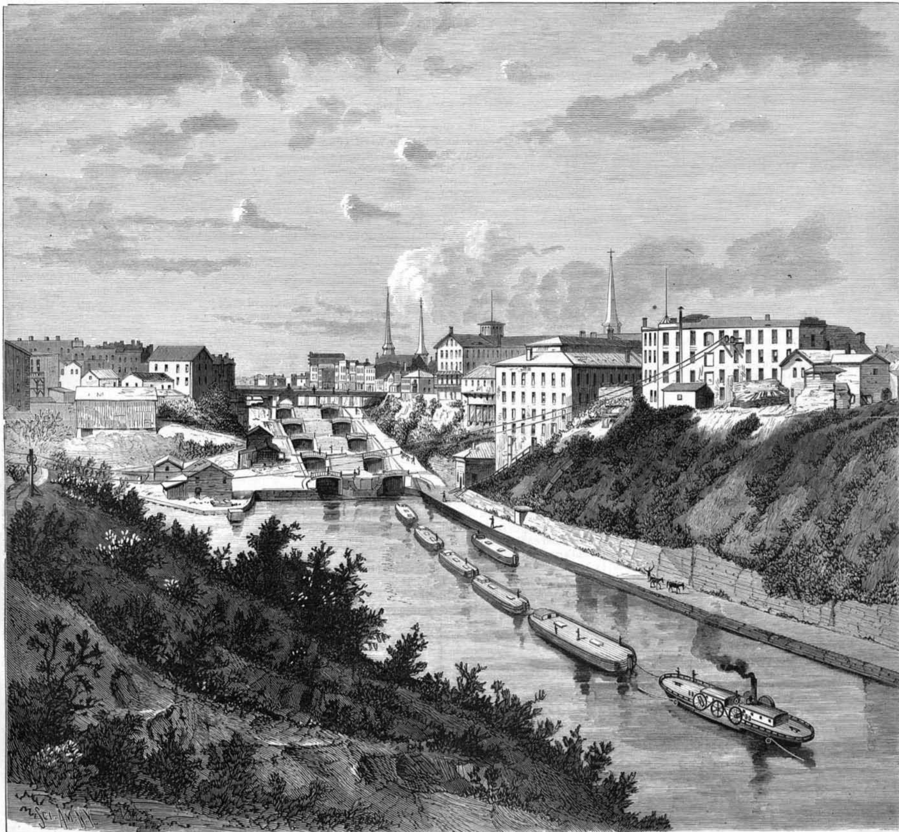
THE BELGIAN SYSTEM OF CABLE TOWING.—THE LOCKS AT LOCKPORT, N. Y.
