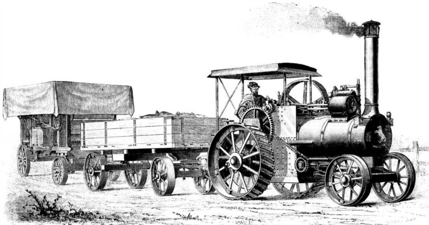
AVELING & PORTER'S ROAD AND FARM LOCOMOTIVE AND TRAIN.
