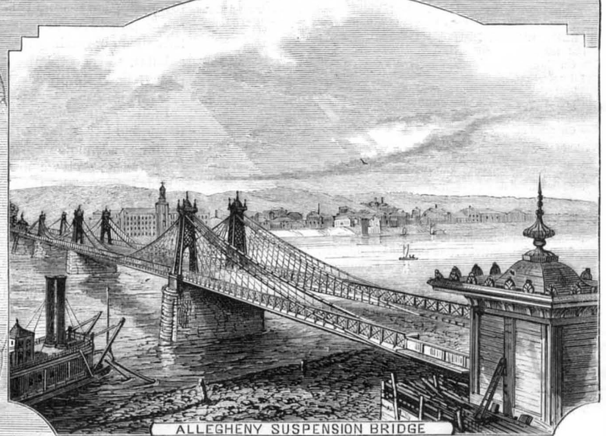
ALLEGHENY SUSPENSION BRIDGE
