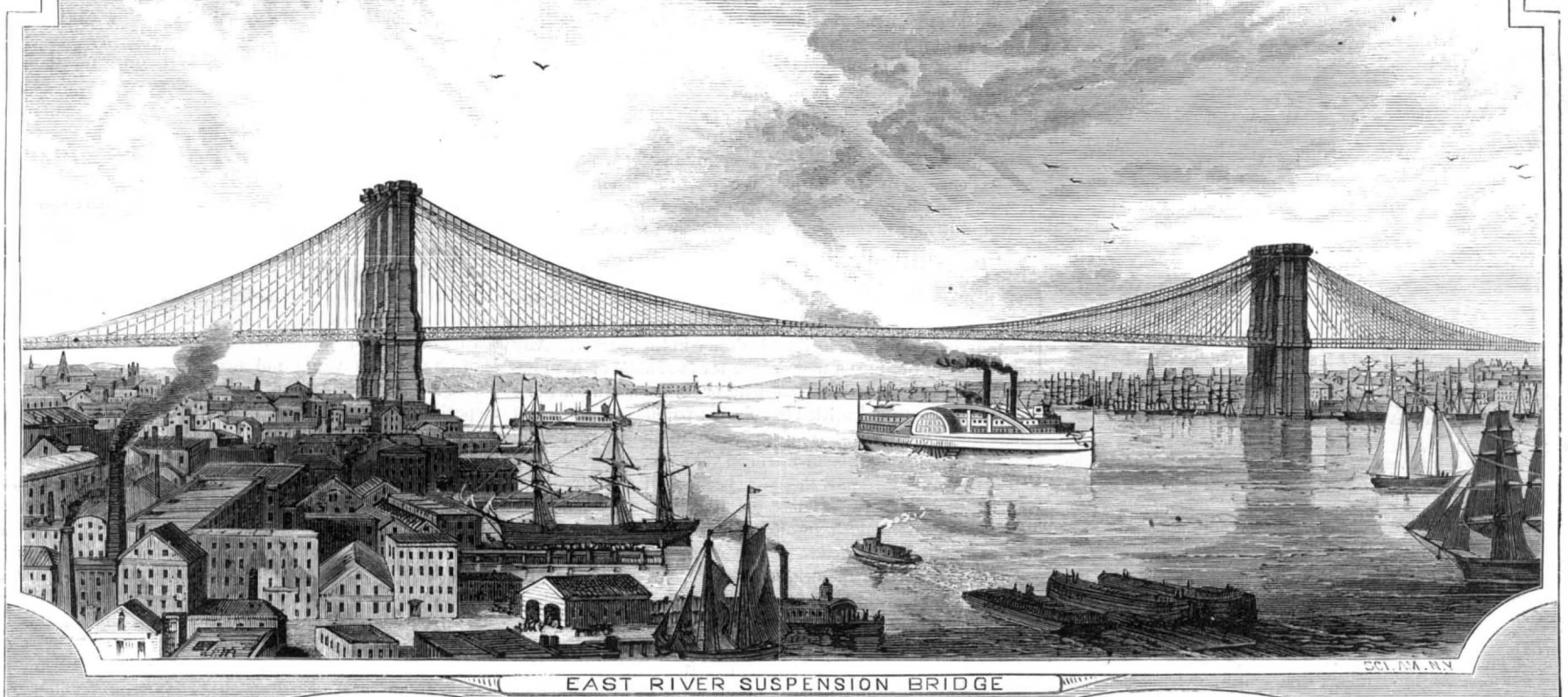
EAST RIVER SUSPENSION BRIDGE
