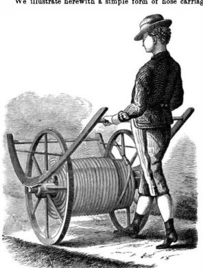
adapted to carrying hose from point to point for watering gardens, washing sidewalks or carriages, extinguishing fires, and many other purposes. The invention is so plainly shown in the engraving that little explanation is needed. It consists of a reel journaled in the curved frame, the rear bar of which serves as a handle. When disposed as represented, with a coil of 200 feet of hose, it can be moved by a child, and forms a very light, useful, and convenient ment pour l'Industrie Nationale.
