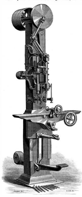
cally reciprocated chisel has obtained a preference. Other systems, such as rotating tools of various designs, are in use for special purposes where the same results could not be produced, or the stuff be conveniently handled, with the reciprocating mortising machine.
