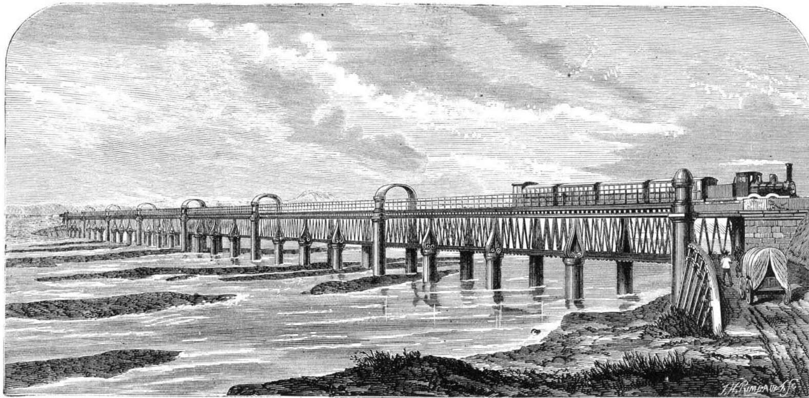
BRIDGE OVER THE WAITAKI NEW ZEALAND.
