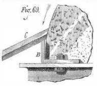
The handle in which the graver is held should be sufficiently long to enable the operator to grasp it with both hands and thus to hold it steadily, even though the work may run very much out of true. For use on wroughtiron, the flat hand tool.
