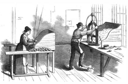
Fig. 2.—PRESSING AND TURNING SMALL WARE.
