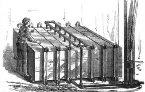
Fig. 4.—PRESSING THE WATER FROM THE SLIP.
