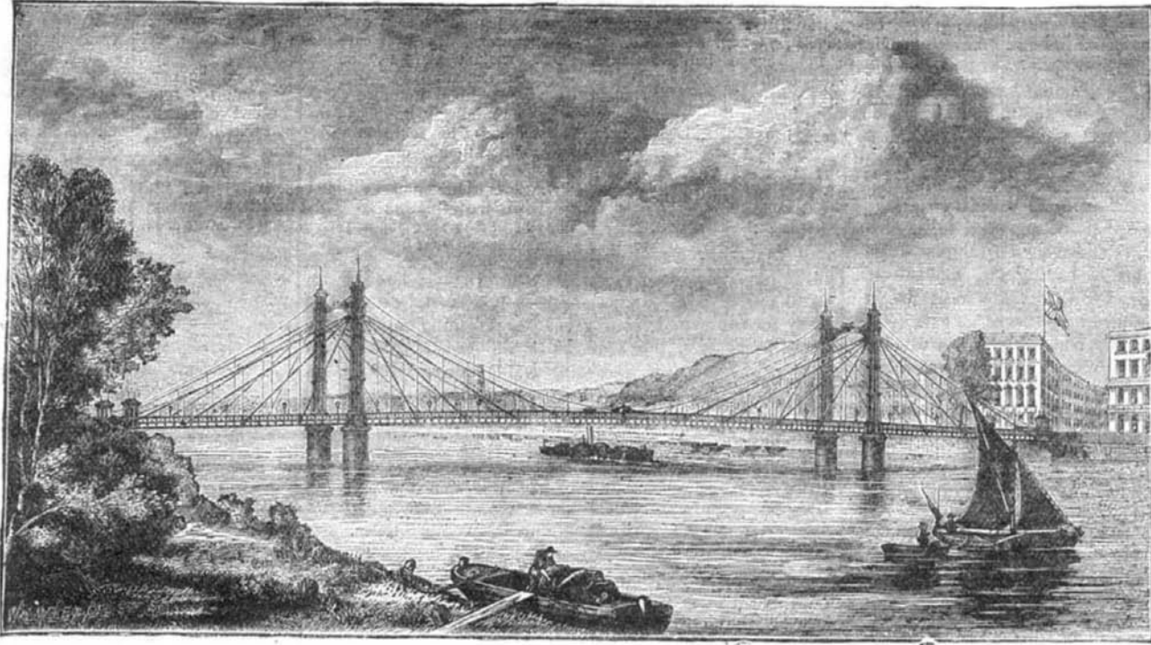
THE ALBERT IRON BRIDGE, LONDON, ENGLAND.—Fig. 1.
