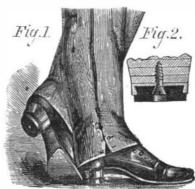
Dr. Batwell states that the invention has been fully tested, I a diameter to fit within a flange on a metal plate and to pro ject below the same, forming a wearing surface of the heel. This is attached by a fastening screw and a conical metal washer formed to fit the under side of the screw head. The latter is forced into the disk, which it pushes into the dovetail flange by which it is securely held. As the wearer turns upon his heel, the plate will partially revolve and change its
