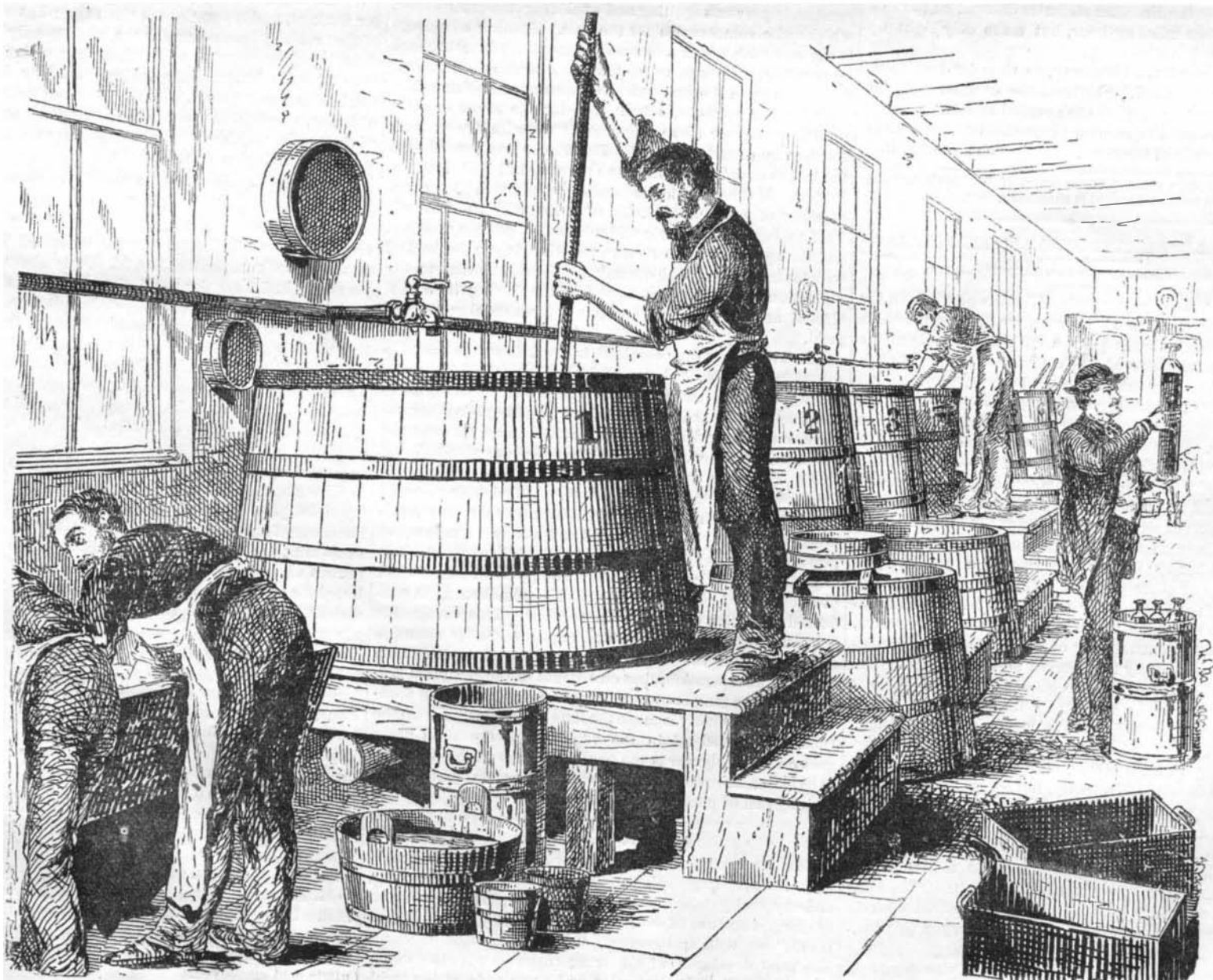
MANUFACTURE OF ARTIFICIAL BUTTER IN NEW YORK.—THE STEAMING VATS.
