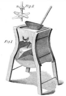
C. is used merely to close the slit in the cover of the churn, to prevent the cream or milk from being dashed out. A plate, D, adjustable with a set screw, is secured to the handle to prevent the hand from sliding down. This swinging motion allows a given amount of agitation to be given to the cream or milk, with less fatigue, probably, than is caused by any other kind of motion, from the relation of the resistance to the muscles which overcome it.
