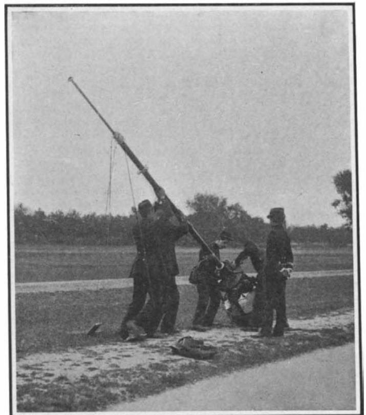
Erecting the telescoping mast.
