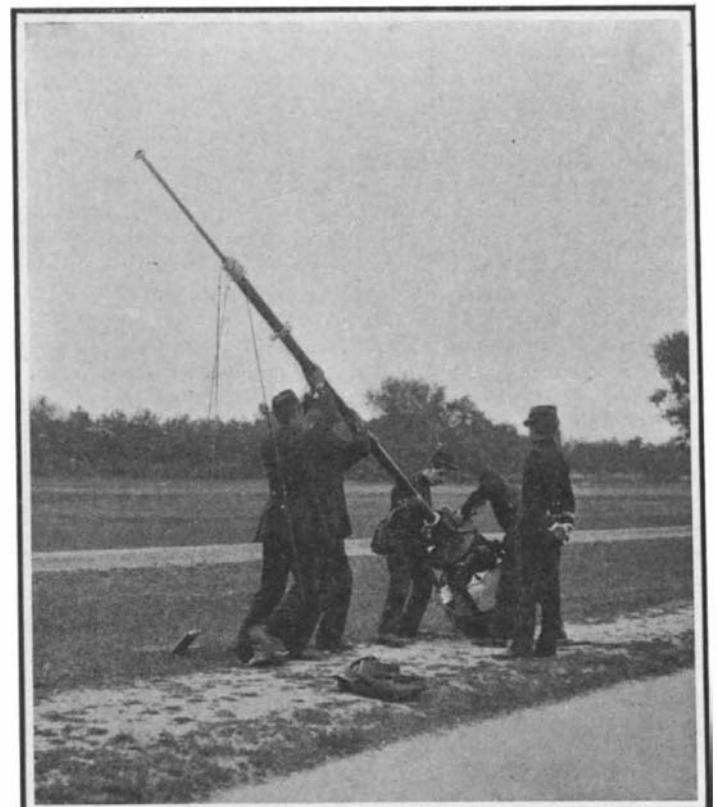
Erecting the telescoping mast.
